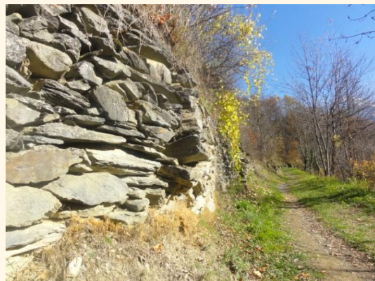
The stone walls start falling apart
