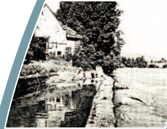
The turbines of the factory at the site of the Serre Water Mill, Feugier-Sappey
