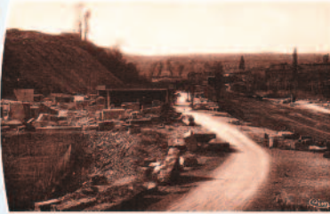
Porcieu, A building site and the Fontaine Blanche station, An Old Postcard
