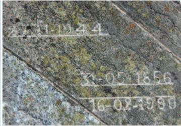
Water level marks engraved onto the wall of the bridge at Sault-Brénaz
