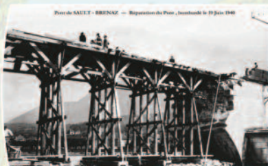
Repairs of the sabotaged bridge in 1940, old postcard
