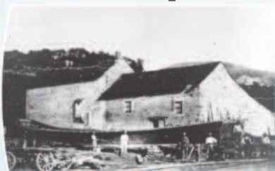
The construction site Chante Merle at Sault-Brenaz, Old Postcard
